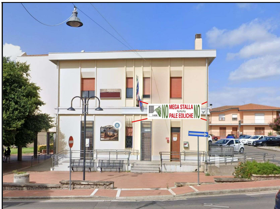
Figura 1: Palazzo Comunale, fronte via Umberto I. L = 5,0 mt – h = 4,0 mt
